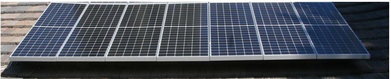
Seven 400W Q Cells Q.PEAK DUO L-G5.2 deployed on a rooftop
